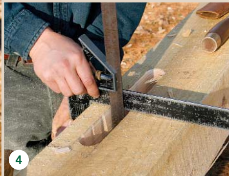
Wedged dovetail Tie beam-post
