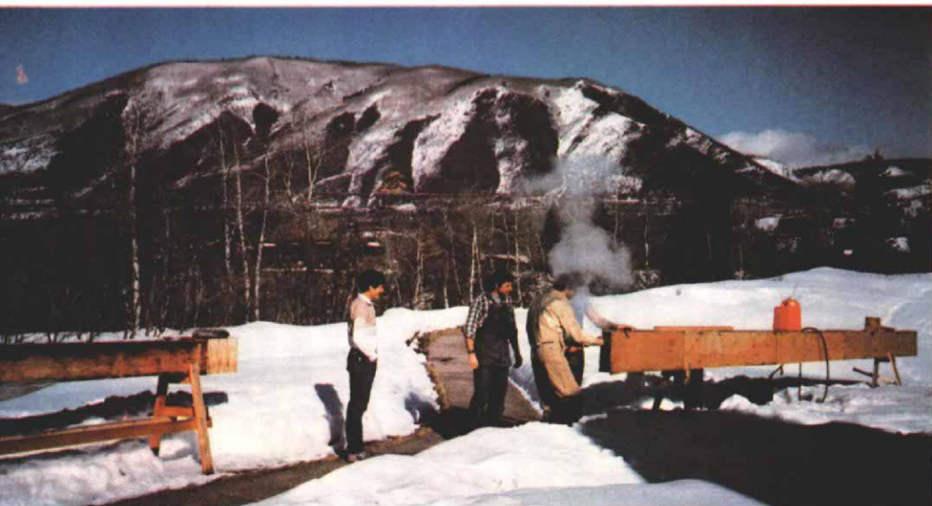
The twisting curves in this stair are so severe that even the thin laminations had to be steamed before they were pliable enough to bend around the forms.
