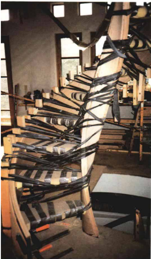
Truck-tire inner tubes, cut up and laced into long bands, were used to clamp the final layer of cherry in place while the epoxy set.
