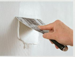
**Scrape it off.** Pull the compound off the wall. Keep the knife tight; the first coat should fill only the mesh. Cover the entire wall, keeping this first layer tight to the mesh. Let the first coat dry, then lightly sand and recoat in the same manner.
