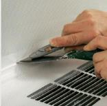
**Trim to fit.** Use a taping knife and a utility knife to trim the mesh around the casing, the baseboard, and the ceiling. Press the mesh into the joint, then trim it with the knife.
