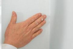
Overlap, but give it room. Overlap the next piece, holding it back from the corner about ½ in. Keeping the overlapping edge away from the corner will ensure that it won't be snagged when joint compound is applied. Wrap outside corners the same way.
