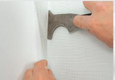
Lap, don't butt. Butting two pieces into an inside corner will result in cracks over time. Instead, run the mesh about 2 in. past the corner. Smooth it out to remove wrinkles, then go back and tuck it tight into the joint using a 6-in-1 tool or a taping knife.
