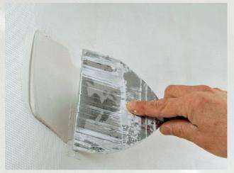
**Use a side stroke.** Using a 5-in. taping knife, apply the compound to the wall with a side-to-side stroke. Be sure not to lift the mesh where it overlaps and where it has been trimmed.
