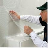
Keep it smooth and straight. Use your hand to press and smooth the mesh onto the wall. Peel back the fabric, and reposition it as needed to remove wrinkles. Overlap each section by 1 in. to 2 in.
