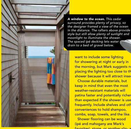
The spaced ipé decking lets water drain to a bed of gravel below. want to include some lighting for showering at night or early in the morning, but Mark suggests not
