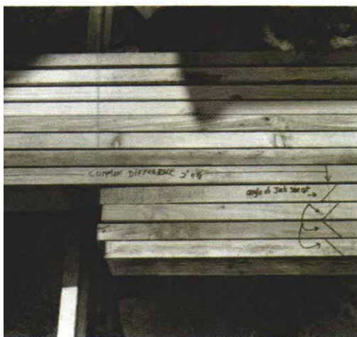
Jack rafters stacked on a rafter bench show the common difference of 2 ft. 4 \frac{7}{8} in. on an 8-in-12 pitch using a 24-in. spacing. The diagonal lines indicate the direction of the side cut that will produce pairs of jacks (left and right) for each hip rafter. The bird's mouth and tail will be marked with the common-rafter layout tee.
