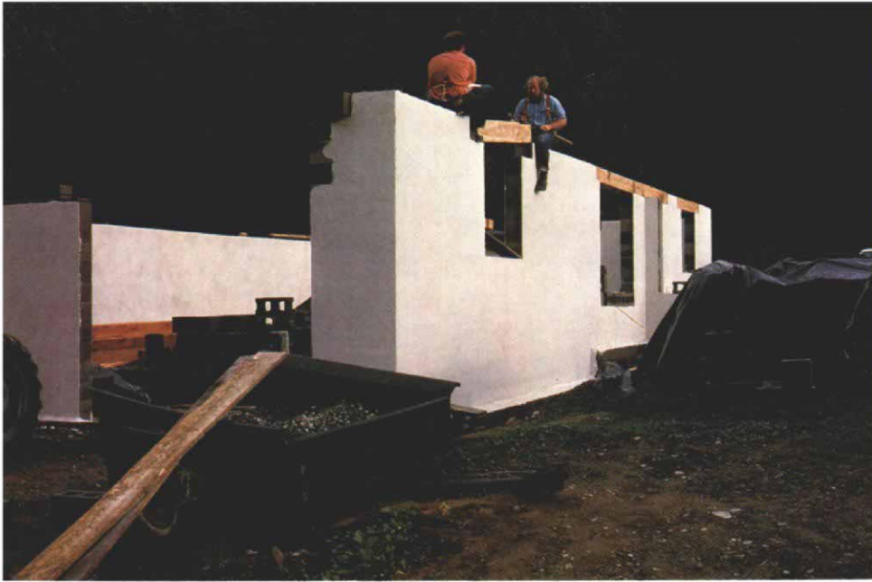
The first course of block is laid and leveled in mortar, as at right. The corners are built up three courses, then a level line is strung between corners. Dry block fills in up to it. Shims are used where necessary to keep blocks aligned. A mason's corner block, which holds a level line that is also the correct plane for the face of the blocks, is visible on the second course. Once the walls have been built up around openings, headers must be installed. These can be steel, concrete or wood, as above.
