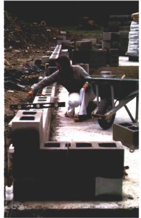
The first course of block is laid and leveled in mortar, as at right. The corners are built up three courses, then a level line is strung between corners. Dry block fills in up to it. Shims are used where necessary to keep blocks aligned. A mason's corner block, which holds a level line that is also the correct plane for the face of the blocks, is visible on the second course. Once the walls have been built up around openings, headers must be installed. These can be steel, concrete or wood, as above.
