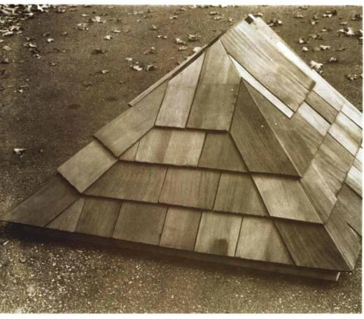
are not sufficiently offset from joints between other shingles. Cut some 2-in. by 8-in. strips of flashing out of zinc, aluminum or copper, and slip them under the splits.
