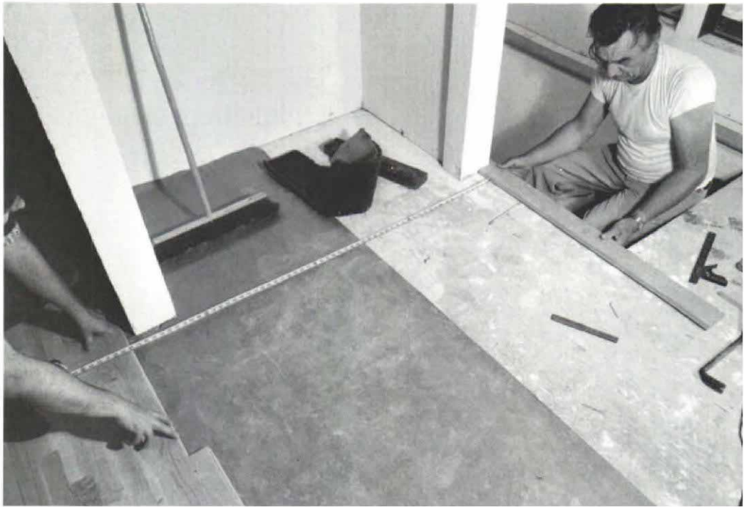
The distance from the advancing floorboards to the stairwell nosing is measured to check for parallel, above. Once this is established, the nosing is cut to length and screwed in place. In the finished floor, below, the strip next to the angled nosing piece required notching. The nosing was removed to let in the strip, then replaced. The countersunk screw holes were plugged.
