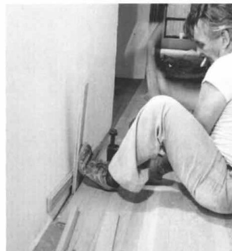
The last course. Strips are levered into place, above, and face-nailed with a power nailer.
