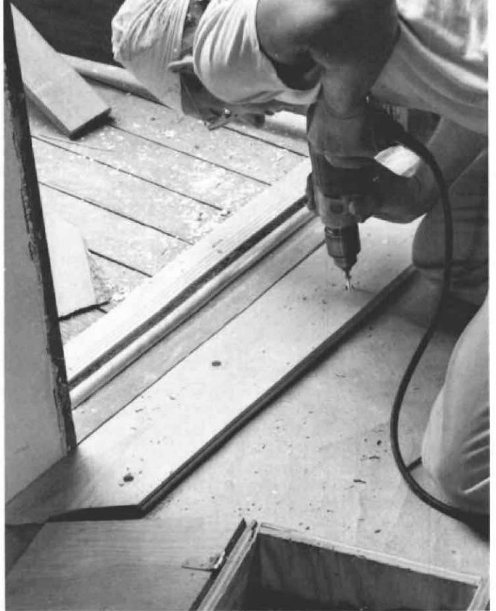
At a doorway, a header board is screwed in place 8 in. o.c. with #10 2-in. square-drive screws. Hardwood plugs, with their grain turned at 90° to the grain of the header board, will fill the counterbores. The first course of flooring will be mitered to meet the edge of the header board.
