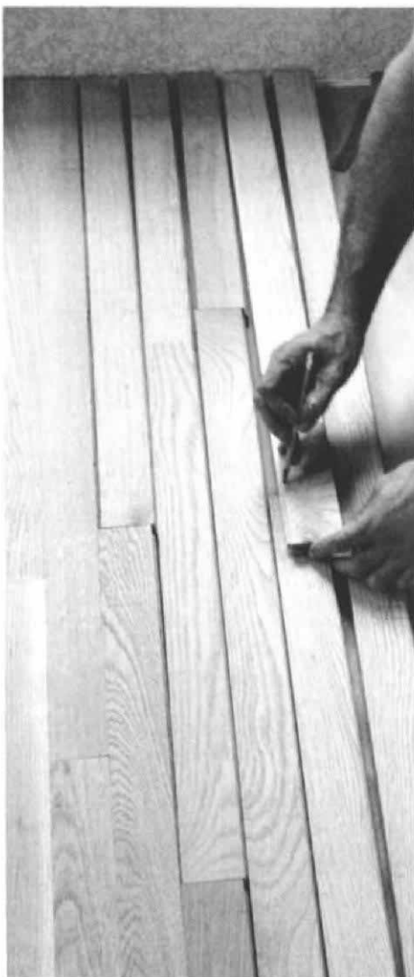
Two header boards intersect in a mitered corner. The door casing has been trimmed off at the bottom to allow the flooring to slip under for a finished look. The tape measure registers the distance from the board's face edge to the baseline.
