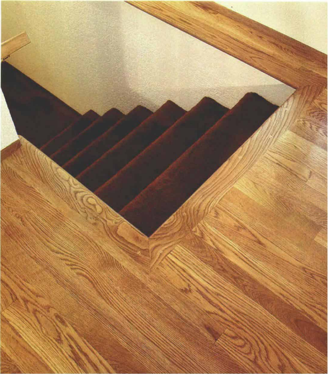
The distance from the advancing floorboards to the stairwell nosing is measured to check for parallel, above. Once this is established, the nosing is cut to length and screwed in place. In the finished floor, below, the strip next to the angled nosing piece required notching. The nosing was removed to let in the strip, then replaced. The countersunk screw holes were plugged.
