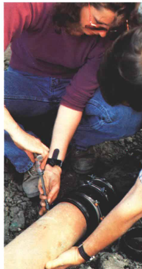
Cast-iron and clay waste lines are connected with a Calder coupling. A thick bushing fits over the smaller pipe to equalize the different outside diameters.
