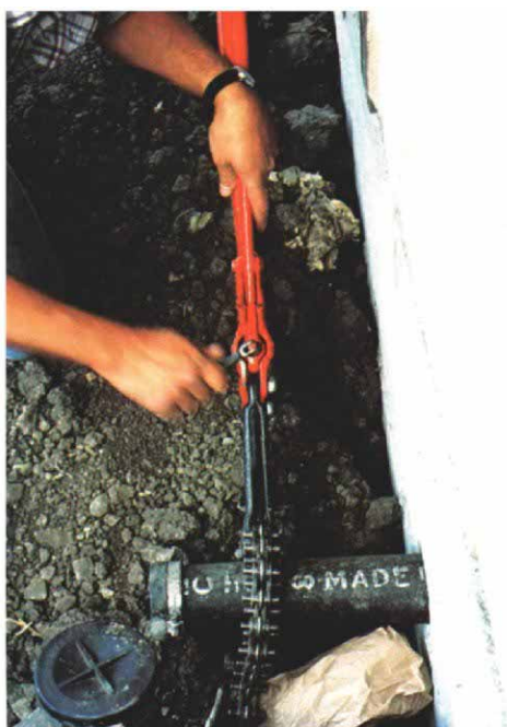
A snap cutter is used for cutting cast-iron drain, waste and vent (DWV) pipe or clay-tile sewer pipe. Integral cutters break through the pipe as the chain is tightened. In this photo, a plumber is adjusting the tension of the chain before snapping the pipe by bringing the scissor handles together.
