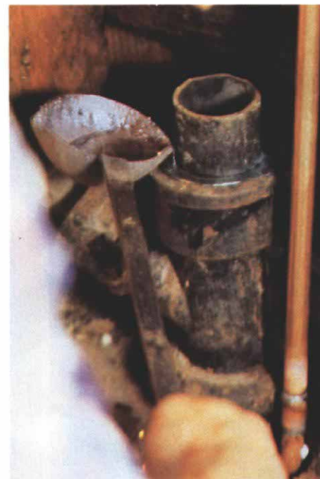
Adding drain, waste and vent lines. Most new DWV lines are plastic, but in old houses, they need to be joined to existing cast-iron pipe. At left, lead is melted with a torch, then poured around the oakum-packed joint between the cast-iron bell housing and nipple of the waste line, above, to seal it. Then a plastic sanitary tee fitting will be plumbed onto the cast-iron nipple with a no-hub coupling. A neoprene sleeve will seal the joint.
