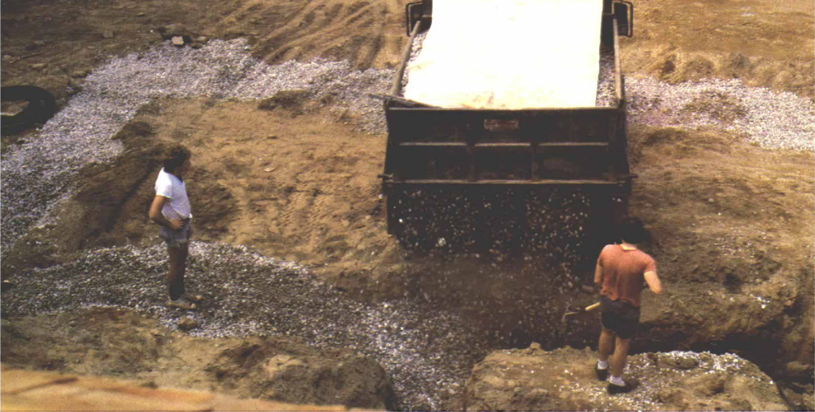
Washed stone is dumped straight from the truck into the foundation and outlet trenches.
