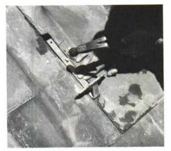
Snow guards. Nailed to the roof lath between slates, these aluminum or cast-iron elements are designed to hold snow on upper sections of the roof, preventing damaging ice and snow accumulation at the eaves. One slate should be notched to fit around the mounting strap, as shown above. The following course covers most of the strap (facing page). Once you master the nailing technique, a roof with no hips or valleys can be slated quickly.
