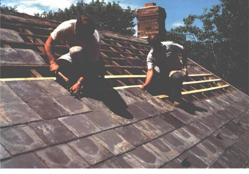
them are Glendenin Bros, Inc. (4309 Erdman Ave., Baltimore, Md. 21213), Prudential Metal Supply Corp. (171 Milton St., East Dedham, Mass. 02026.) and Vermont Structural Slate (Box 98, Fair Haven, Vt. 05743). Correct nail length for standard ¾6-in. slate is 1½ in., for either copper or galvanized nails.
