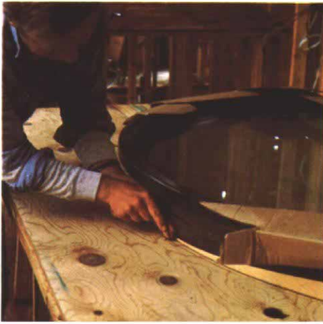
Using the dormer's window as a pattern for the arched header, above, Phelps traced its shape onto a sheet of \frac{3}{4} -in. plywood. Once it was cut out, he used it as a template for six more plywood layers, which were all then glued and screwed together to form the header, right.
