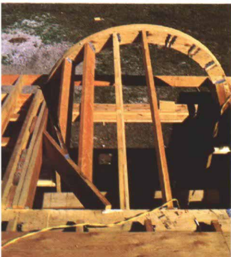
To approximate the half-ellipse, Phelps installed two 2x10 headers on each side of the rough opening, below. The inside corners were blocked to produce the curve. The dormer is covered with Veral, a roofing system that consists of copper foil bonded to glass-reinforced asphalt. Workers roll the material out and join sections by melting the asphalt, right.
