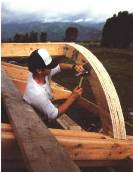
To approximate the half-ellipse, Phelps installed two 2x10 headers on each side of the rough opening, below. The inside corners were blocked to produce the curve. The dormer is covered with Veral, a roofing system that consists of copper foil bonded to glass-reinforced asphalt. Workers roll the material out and join sections by melting the asphalt, right.
