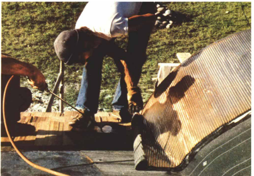
To approximate the half-ellipse, Phelps installed two 2x10 headers on each side of the rough opening, below. The inside corners were blocked to produce the curve. The dormer is covered with Veral, a roofing system that consists of copper foil bonded to glass-reinforced asphalt. Workers roll the material out and join sections by melting the asphalt, right.
