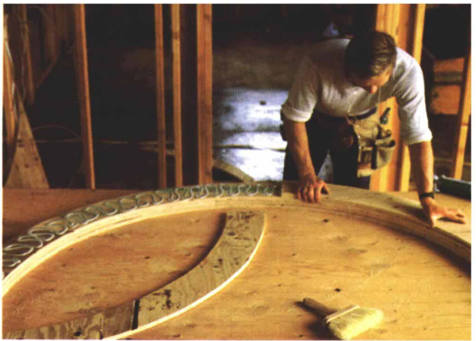
Using the dormer's window as a pattern for the arched header, above, Phelps traced its shape onto a sheet of \frac{3}{4} -in. plywood. Once it was cut out, he used it as a template for six more plywood layers, which were all then glued and screwed together to form the header, right.
