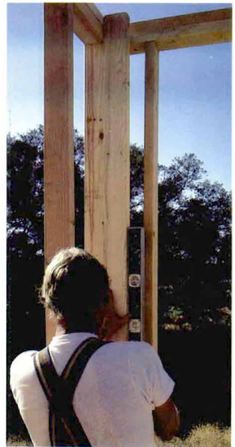
Plumbing. The length of the level you use is a lot less important than being sure that it is dead-on accurate. Here a 4-ft. level is attached to a straight stud with bent-over nails. Using 1x spacers at the top and bottom of the stud (or manufactured aluminum spacer blocks on an 8-ft. level) will ensure an accurate reading despite bowed wall studs.
