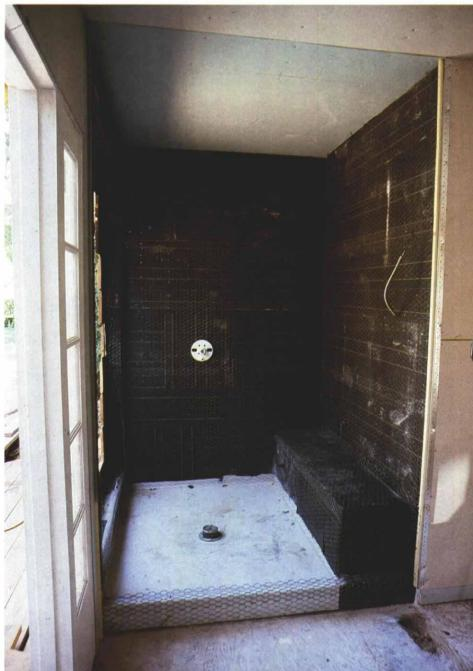
**Water test**—Except for placing the screeds, the job is now ready for floating the mortar bed, but at this point, do a water test. Plug the lower drain and fill the pan with water right to the top of the curb and let it sit, undisturbed, for 24 hours. If possible, get under the floor with a flashlight and look for any sign of leaks.
