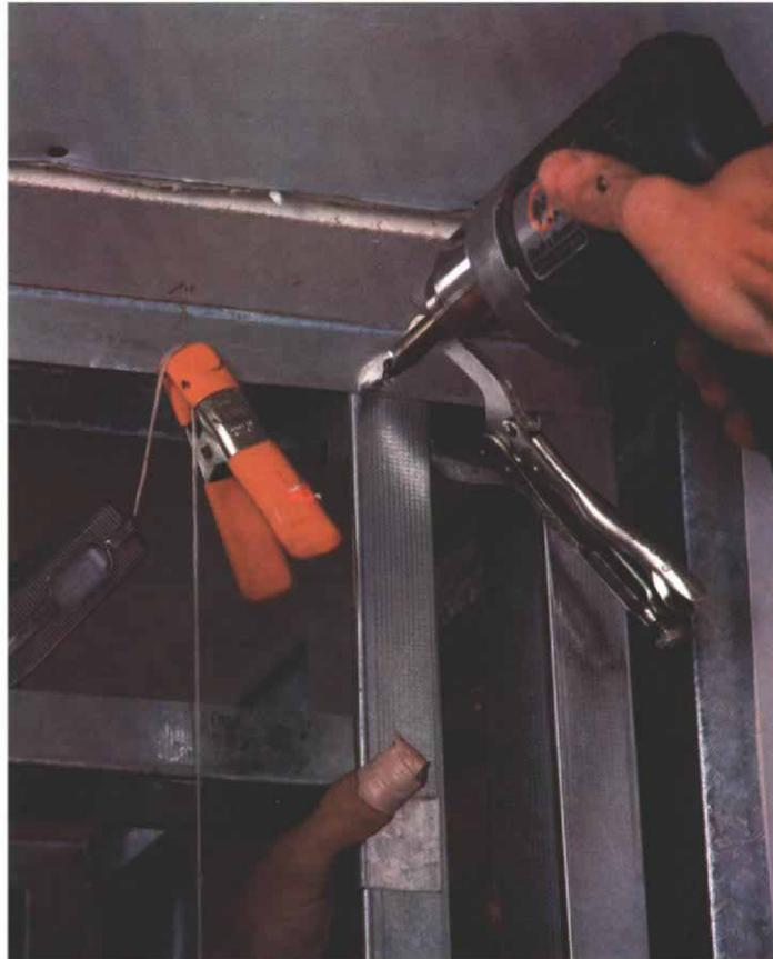
**The workhorse tool for installing light-gauge steel framing is the screw gun or reversing drill. Locking C-clamps hold stud and track together until the screw is run home, while a spring clamp anchors a plumb line.**
