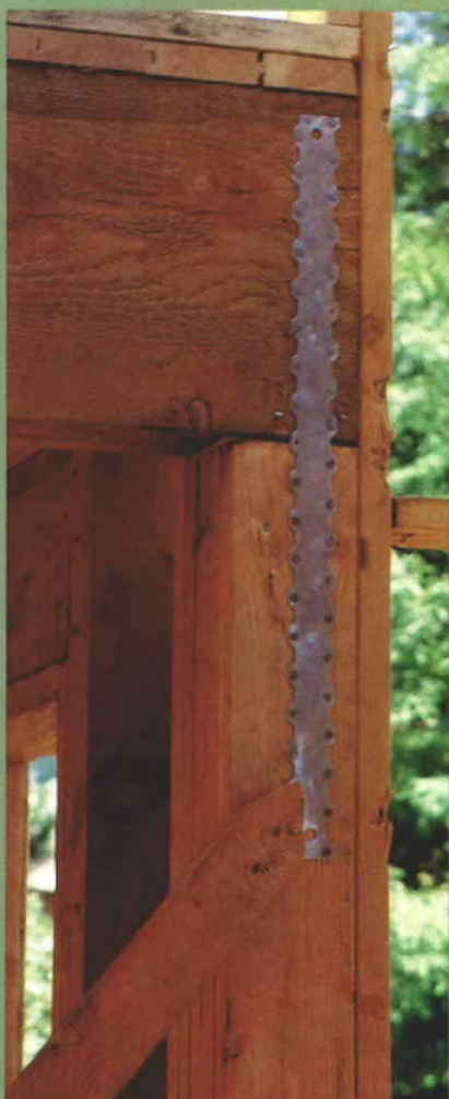
Steel straps are useful tension ties throughout wood-frame buildings. Here a steel strap is used to resist the uplift load on a beam.
