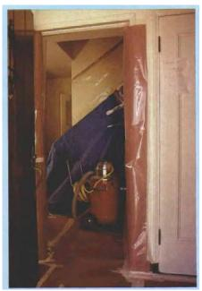
Gerstel protects floors with a double layer of kraft paper, and walls with polyethylene sheeting stapled to wood strips. If walls and ceilings are to be removed, he puts down a layer of plywood on top of the kraft paper, and duct-tapes the seams.
