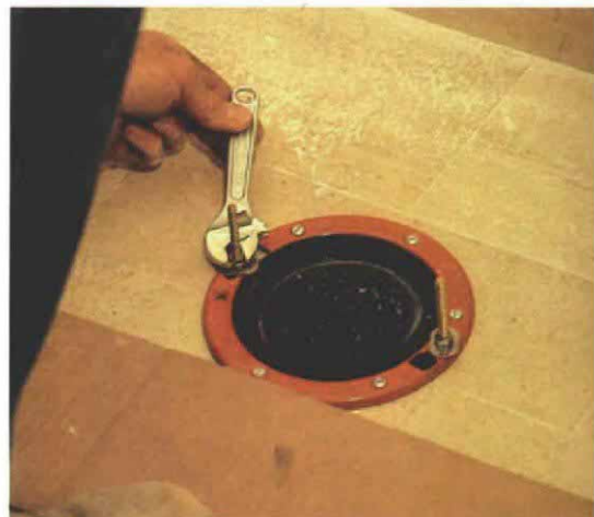
3. Slots in the steel ring of a closet flange accept closet bolts. They will protrude through holes in the base of the toilet.
