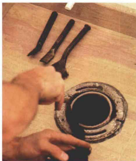
6. Skaates uses a yarning iron to push the oakum into the space between the cast iron closet flange and the drain. Next he will use a packing iron (the right-hand tool in the trio above) to press it home.
