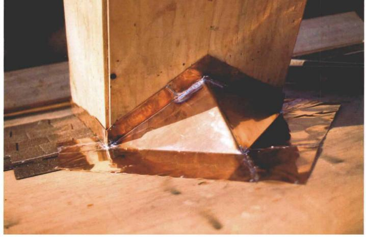
Building and flashing a cricket are the same whether for a masonry chimney or for a wooden chimney structure like the one above, which houses a pair of woodstove chimney pipes. Other metals will work for the hashing, but copper is the easiest to solder.
