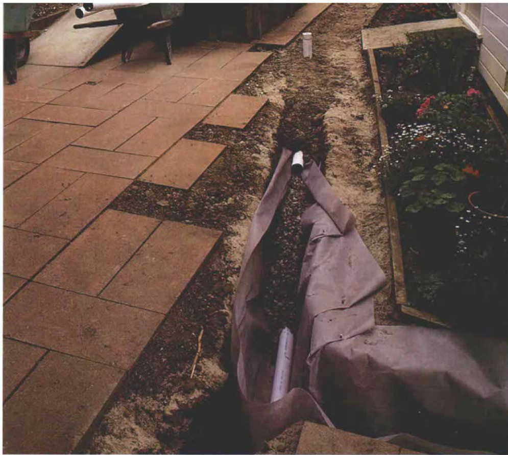
Two pipes. To properly drain a structure, you need to pick up subsurface water moving through the soil as well as runoff carried from flat surfaces and roofs. The pipe in the bottom of the trench above is perforated, with its holes oriented downward. Gravel covers it to within a foot of grade, and filter fabric is folded over the gravel to keep fines from clogging the drain line. The top pipe carries surface runoff from downspouts and drains. The pipe stub projecting above the tamped earth will attach to an area drain.
