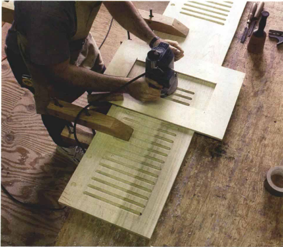
With a shop-built jig and a \frac{5}{16} -in. core box bit in a plunge router, the author cut the vertical flutes that create the frieze under the mantel shelf (photo above). Where the joint would show between the horizontal and vertical members of the frame, the pieces are mitered (photo below). The butted portion will be hidden behind the pilaster. Notice how the ends of the flutes are carved so that they appear to point upward. (Photo below by author).
