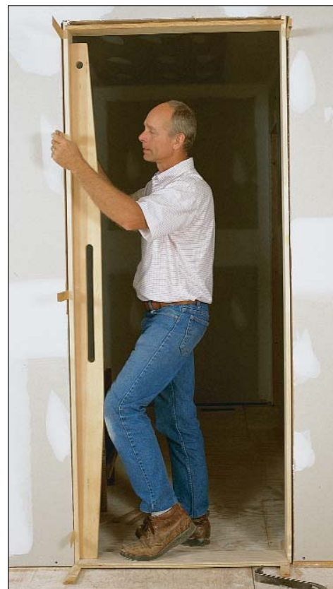
The tapered edge of this straightedge fits the author's knee height. The taper on this 6½-ft. straightedge begins 19 in. from the end so that the author can hold it against a door jamb with his knee while he inserts shims.
