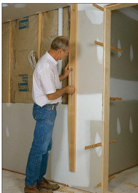
Checking the straightedge. Draw a line on a wall on one side of a straightedge; then flip the straightedge and hold it to the line. If the edge is straight, it will line up with the pencil mark.
