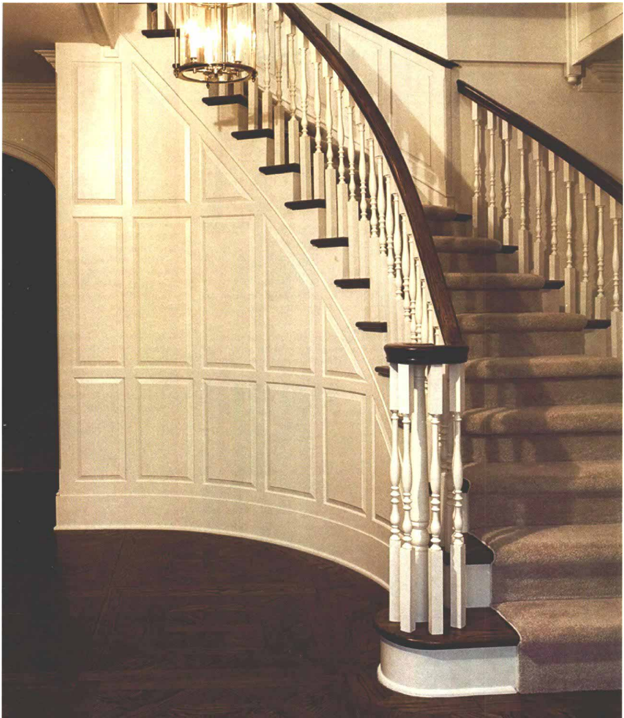
The traditional look is made of nontraditional methods. By building up layers of different materials, including bending plywood, pine moldings and tempered hardboard, Glenn Bostock duplicated the look of a traditional frame-and-panel wall.
