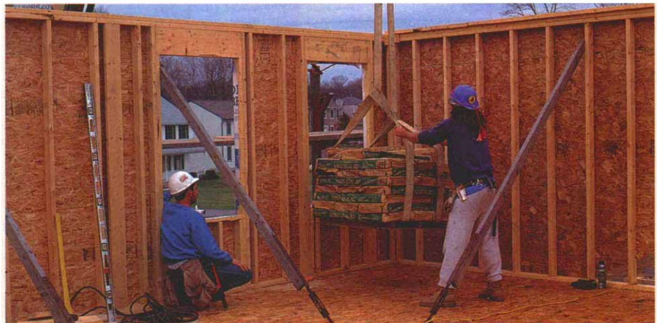
Roof shingles are dropped near a window. The crew member on the left signals the crane operator while the other crew member guides the pallet of shingles to its temporary home.
