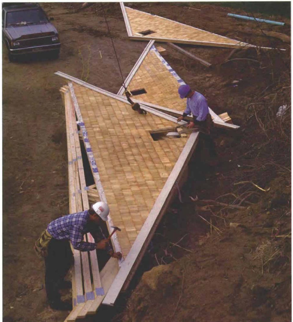
Nails for attaching the gable truss are started on the ground. To facilitate setting the gable truss, nails are started along the bottom chord. When the truss is in position, a crew member on a ladder will drive the nails into the top plate of the gable-end wall.
