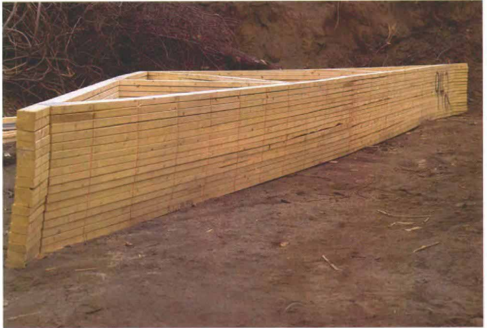
Stacked for easy layout. With the trusses stacked neatly on the ground, layout lines are drawn on all of them at once. The line closest to the tail will be used to position the truss on top of the wall plates. The other lines are for ceiling strapping. The top chords are laid out for roof sheathing.
