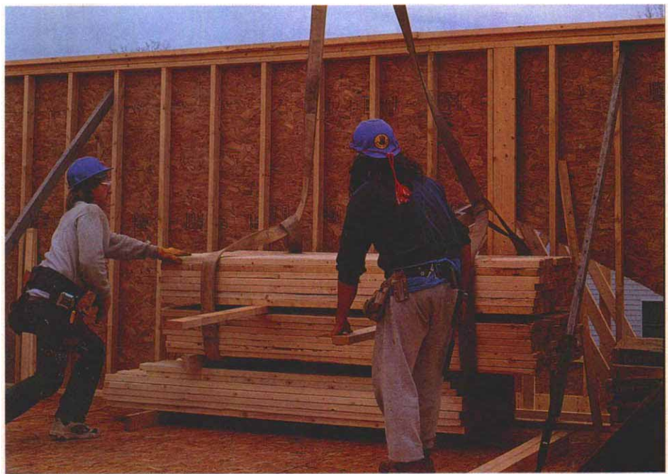
Interior wall framing on the rise. Lumber is stacked ahead of time for an easy crane hoist; crew members land the framing lumber inside the house where it will be out of the way until it's needed.
