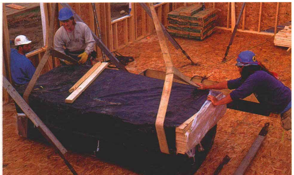
Prepackaged loads of sheathing are easier to handle. The lumber company bundles the sheathing in stacks of 15 to 20 sheets for easy strapping and lifting.
