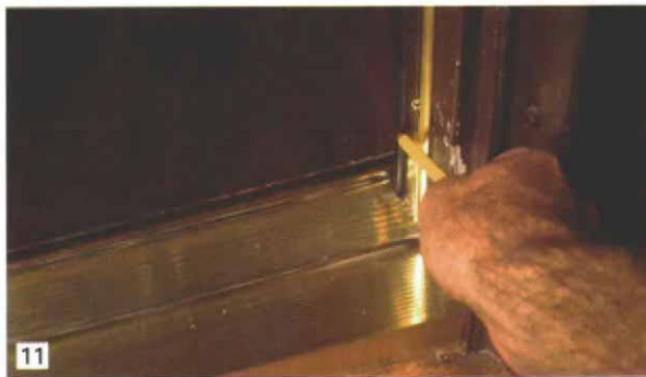
A site-built tool speeds the cut. The author cuts doors with a "shooting stick," a plywood straightedge that has a fence against which he registers the table of his circular saw (10).
