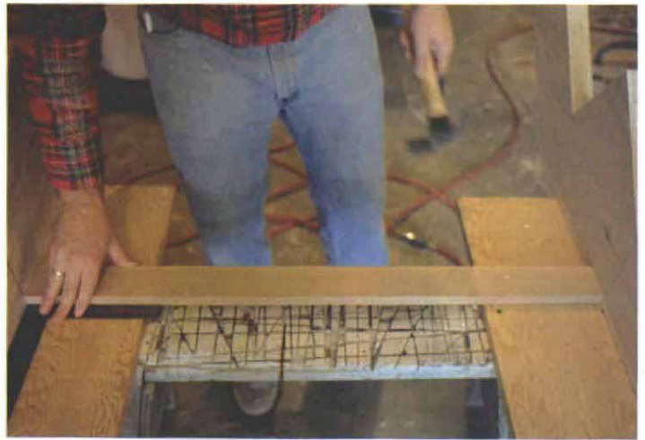
Witness marks help align the stringers in the jig. Lines called witness marks are made with the stringers laid side by side. Then a square and a straightedge align one stringer perfectly with the other.
