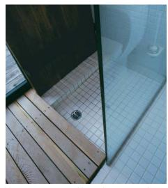
**The duckboards lift up in two sections.** Affixed to sleepers that have been notched for drainage, the cedar duckboards conceal a tile-covered shower pan that has been built into the slab floor.
