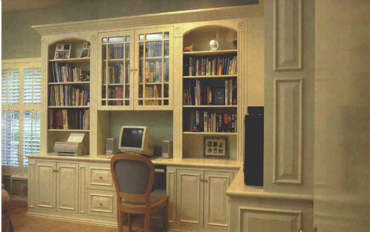
High-quality appearance from a man-made material. Most of the components that make up this cabinet, including the raised panels for the doors, drawers, countertop and cabinet sides, were made from MDF. Once painted, the material is difficult to distinguish from solid wood.
