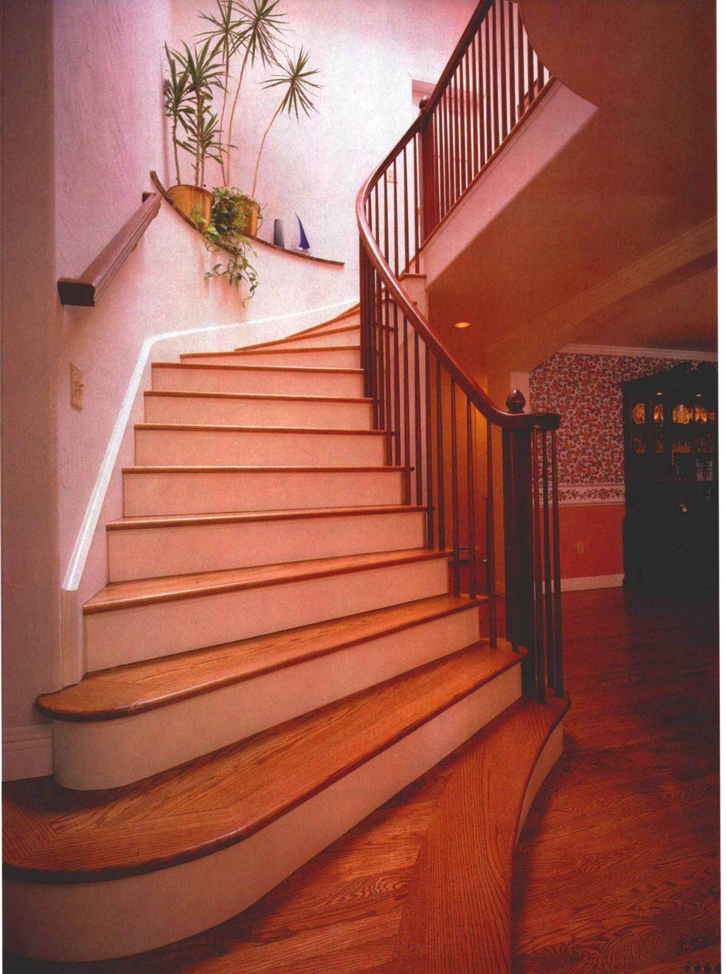
The curves of this finished stair hide its straight skeleton. Built without the rushed panic of gluing a laminated stringer and using methods a journeyman carpenter can master, these stairs look like the product of a master stairbuilder.
