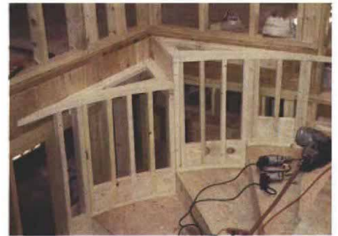
A curved kneewall forms plant shelves. Stepping up with the stairs, this kneewall supports two platforms that will later be used to display plants.
