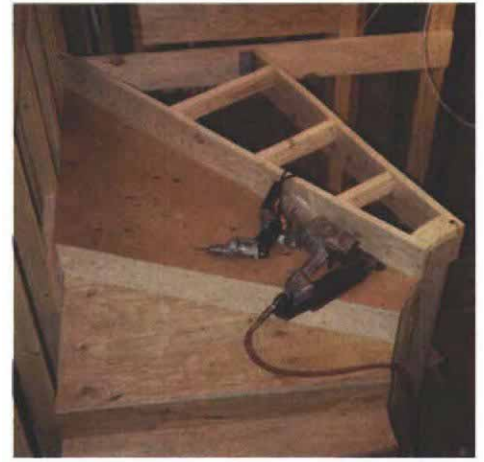
Winding stairs without a stringer. Two-by-tens, resting on the inner wall and fastened to ledgers on the outer wall with framing hardware, support the treads and risers.
