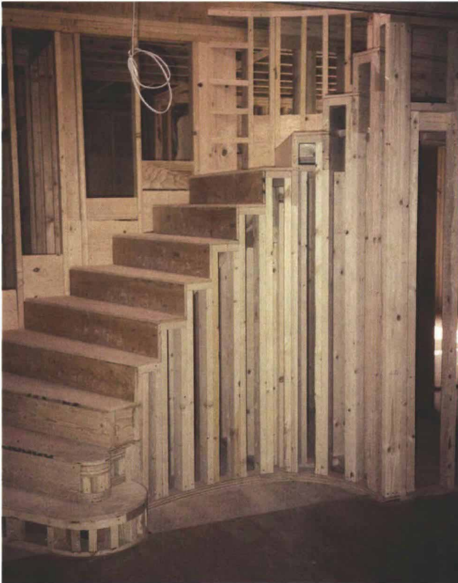
Winding stairs without a stringer. Two-by-tens, resting on the inner wall and fastened to ledgers on the outer wall with framing hardware, support the treads and risers.
