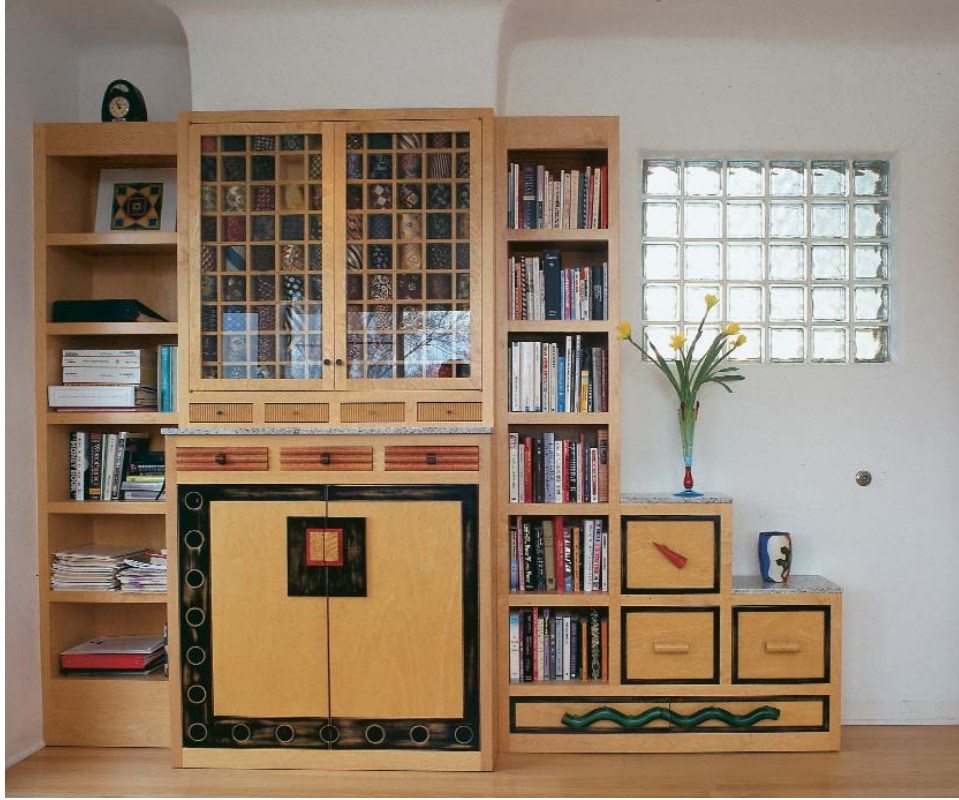
These cabinets are built around the chimney. A full-depth cabinet would have been out of proportion here, but this necktie cabinet is shallow enough to fit the space yet deep enough to have substance. The shelves and drawers that flank it fill out the depth of the chimney. Photo taken at D on floor plan.
