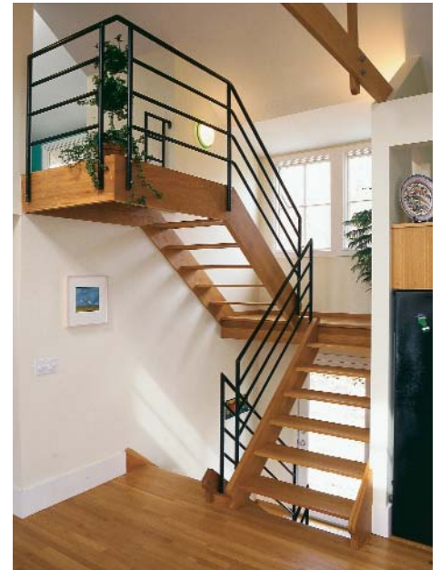
Cantilevered stair leads to an upstairs study. Delicate oak treads, a spare railing and open risers let the light pour through the stair-case. Photo taken at F on floor plan.
