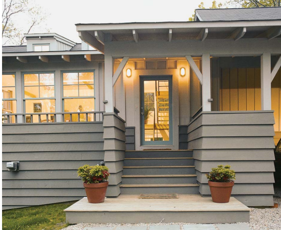
Find the module. An underlying symmetry controls the detailing on the exterior of the house. The battens are on 1-ft. centers to cover the grooves in the T-111 plywood. Windows and their muntins align with the battens. The rafters, on 2-ft. centers, occur over every other batten. Photo taken at E on floor plan.
