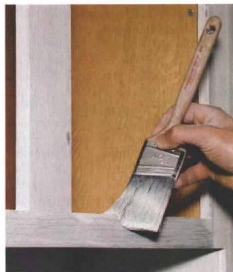
Brushing the cabinet-face frames while the doors dry. The authors start at the inner edge of the frames and work out. The frames are sanded between coats, as the doors are.
