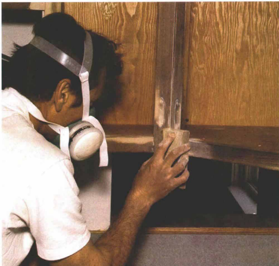
Spackling and sanding are crucial to a good-looking paintjob. Paint highlights surface imperfections, so the authors start sanding with 100 grit and progress to 220 grit before painting.
