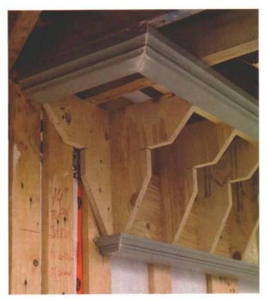
These plywood forms were assembled in 8-ft. sections and screwed to the house. Then the moldings were nailed to the forms, except at outside corners, where they float, nailed and glued only to other moldings.
