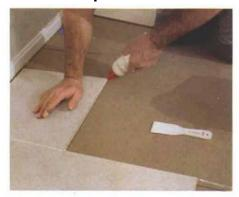
Glue is critical to the flooring's success. Holding the glue bottle at a slight angle is an easy way to control the application of glue. A second bead along the mating tile's edge ensures a tight, waterproof bond. Gaps in the glueline can cause the flooring to fail.
