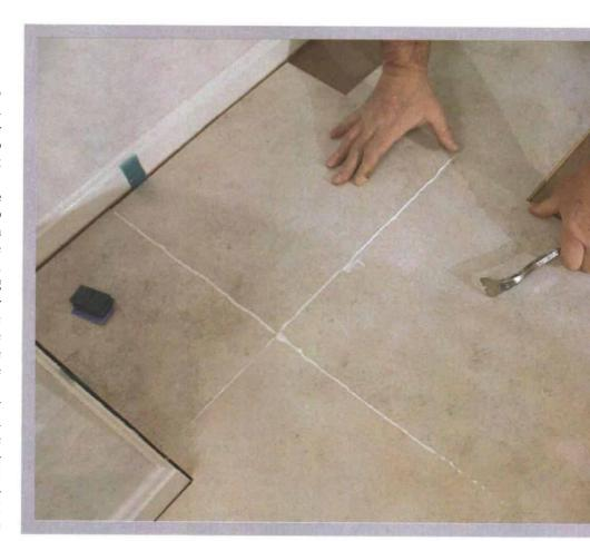
tiles (photo right, facing page). It's important to clean up the glue as you go; if you wait, it becomes more difficult to clean. I inspect the joints when cleaning, too. If a joint is loose, now is the time to tighten it with clamps or blocks.
