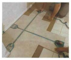
Strap clamps keep joints tight, courses straight. All laminate flooring requires some clamping to tighten glue joints. Specialized clamps can apply pressure over spans of up to 15 ft. or more. As long as the joints are tight, the tile edges will align themselves.
