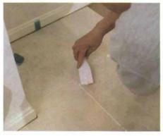
Wipe off excess glue and check the joint. A plastic putty knife makes a good tool to clean excess glue off the flooring. Follow with a damp, not wet, terry-cloth towel; too much water in the towel will dilute the glue and weaken the joint.
