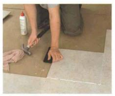
A few careful taps with a hammer and block can close gaps. One way to tighten flooring joints is to use a hammer and a plastic tapping block, which is made to fit the flooring's edges. However, tapping too hard can dislodge other joints.
