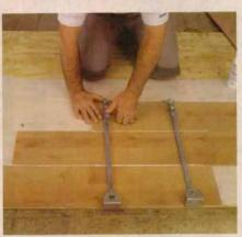
Stagger plank joints when establishing the starter course. When laying plank floors, always build a starter course of three rows, staggering the butt joints by at least the width of the plank. Specialized bar clamps draw the glue joints together.
