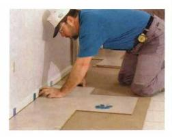
**Dry-fitting the first two rows.** It's important to make cuts and check the fit of the laminate before gluing. Numbering the back of the laminate helps to keep the pieces in sequence. This is also a good time to check for defects.
