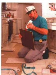
Glue makes laminate flooring work. A special PVA-type glue bonds and permanently seals the surface. The edge-glued flooring floats on the existing subfloor.
