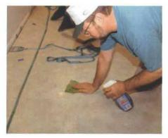
Window cleaner and a towel clean glue haze. After the clamps have been removed, the residual glue haze must be cleaned off before it dries completely. A 1:5 solution of vinegar and water works just as well as the window cleaner.
