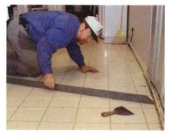
Make sure that the existing floor is flat. After it is cleaned, the floor must be checked for flatness with a straightedge or a chalkline. Any floor deflection of ¼ in. or less over 10 ft. is acceptable.
