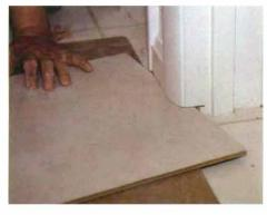
**Checking the fit.** After cutting the door trim and removing the waste with a hammer and chisel, installers make sure that the laminate flooring and underlayment will fit neatly into the space.
