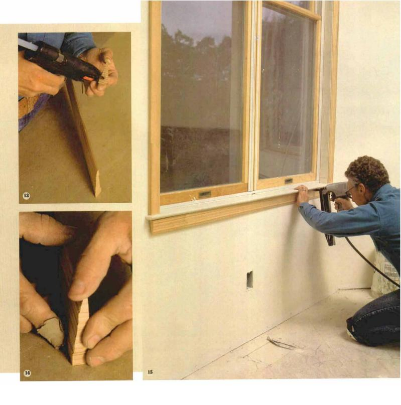
backing here because the screwed connection between the jamb extensions keeps them from being driven out of alignment.
