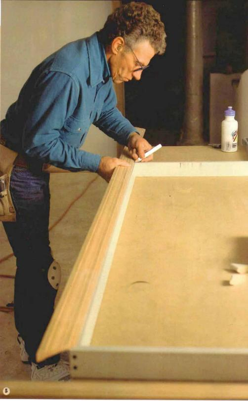
the side extensions. In this case, I measured the window and added  $\frac{3}{16}$  in. for the top reveal, plus  $\frac{3}{4}$  in. for the thickness of the head jamb. The length of the stool (photos 1, 2, 3) depends on the reveals, the width of the side casings and the distance that the stool projects beyond the casing— $\frac{3}{4}$  in. for this job.
