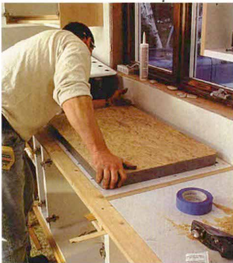
The sink goes here. Built-up layers of flakeboard cut to the sink manufacturer's paper pattern will keep concrete out of the sink opening. Duct tape makes a good moisture barrier.
