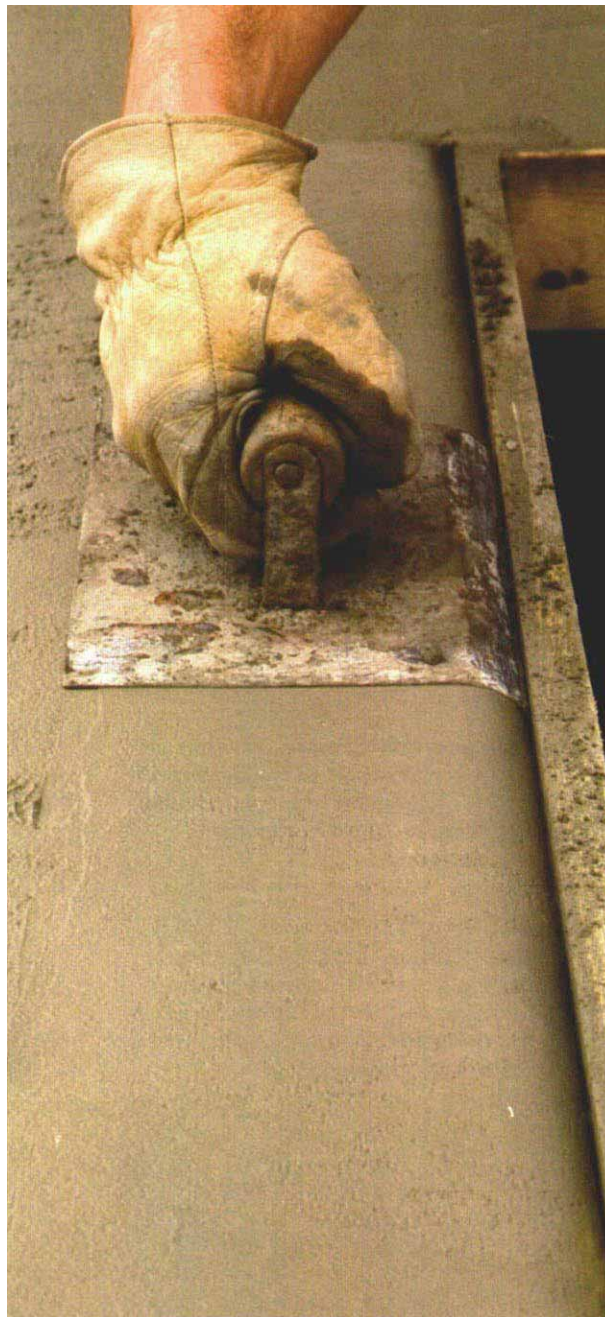
4. A steel edging tool makes a clean radius at the outside edge.
