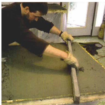
2. Remove the braces, and screed the top.
