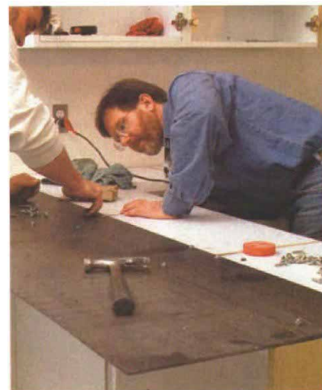
Steel sheet reinforces a wide overhang. Rex Alexander (right) and Mark Story bolt a piece of \frac{1}{4} -in. steel to a cabinet top to support a 10-in. concrete overhang. Bolt heads are inside the cabinets.
