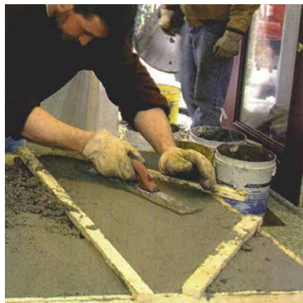
1. Pack the concrete into the forms.
