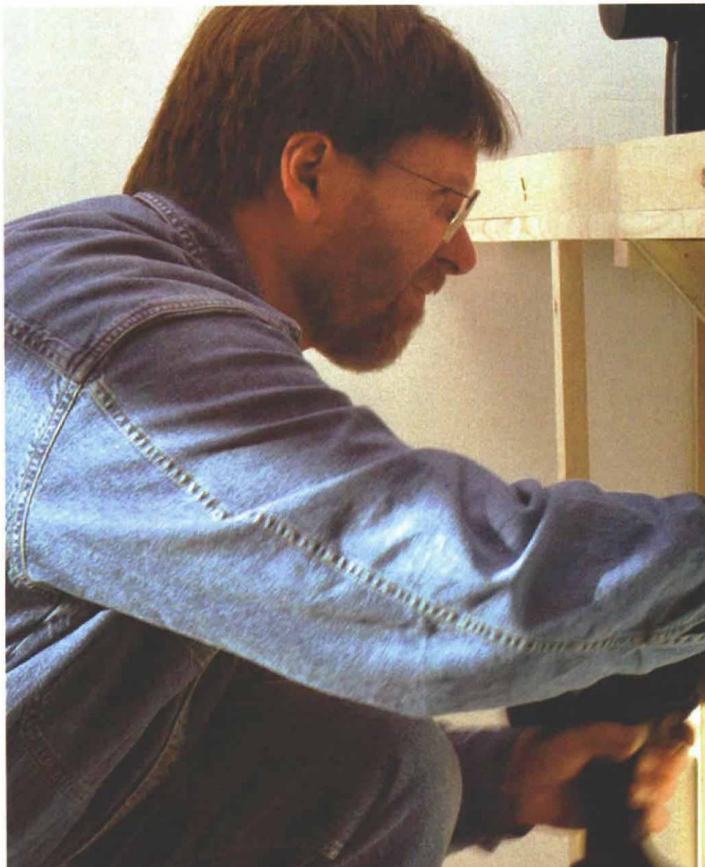
Steel sheet reinforces a wide overhang. Rex Alexander (right) and Mark Story bolt a piece of \frac{1}{4} -in. steel to a cabinet top to support a 10-in. concrete overhang. Bolt heads are inside the cabinets.
