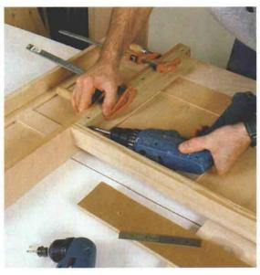
1. Blocking makes a stronger joint. With parts flipped on their backs, the author glues and screws a poplar block at each end of the center panel. Clamps hold the center panel to pilasters while parts are glued and screwed together.
