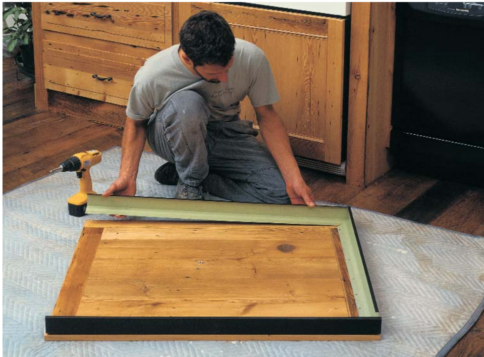
Aluminum channel is the key. Bent into a J-shape, aluminum channel is screwed to the back of the cabinet panel. A gap in the top channel accommodates the refrigerator-door hinge.
