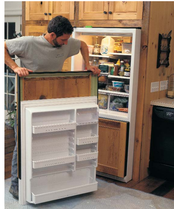
Held in place by gravity and friction. With the door removed, the panel slides easily over the door.
