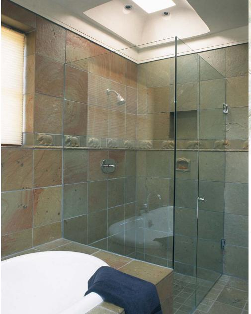
Glass walls are barely there. Tempered-glass partitions, aligned with the grout joints in the tile, neatly corral the shower without making the room feel smaller. Photo taken at B on floor plan.
