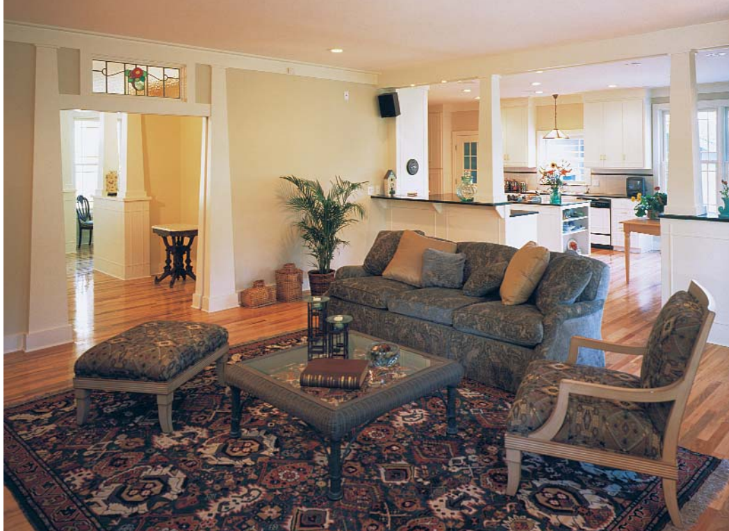
Pocket doors with a theme. To divide the front hall from the family room at the rear of the house, the author inserted a pair of pocket doors below a stained-glass transom light. Door trim resembles a pair of battered columns. Photos taken at F on floor plan.
