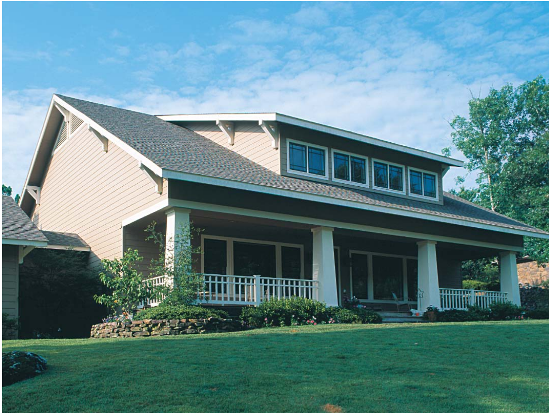
Signature details of a Craftsman-style bungalow. With an inset front porch, beefy tapered columns and knee braces at the eaves, this Arkansas house reflects common architectural themes from the Craftsman bungalow era. Photo taken at A on floor plan.
