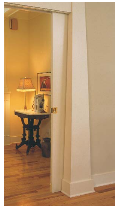
Pocket doors with a theme. To divide the front hall from the family room at the rear of the house, the author inserted a pair of pocket doors below a stained-glass transom light. Door trim resembles a pair of battered columns. Photos taken at F on floor plan.
