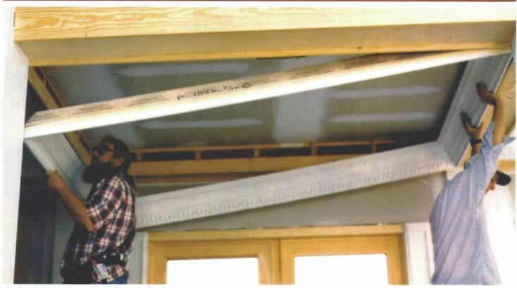
The hardest part is getting through the door. Synthetic crown is so strong yet light that two men can easily lift an entire room's worth into place. Complete preassembly is possible only where walls are less than 12 ft., the maximum length of this molding.
