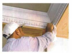
A rag moistened with mineral spirits takes care of squeeze out. Glue that gets on the face of the molding is wiped off before it sets up. Glue that squeezes out and dries can be scraped off with a knife.
