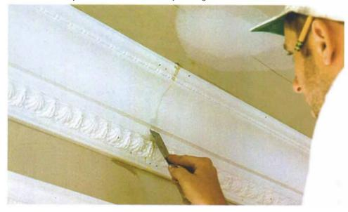
**A little dab'll do ya.** With the miters preassembled and the seams tightly butted, a little bit of Spackle here and there is all it takes to fill in the gaps.
