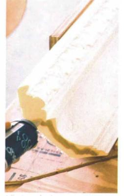
Adhesive makes it permanent. After dryfitting the miter cuts in the setup jig, a  $V_4$ -in. bead of proprietary adhesive (see p. 120) is applied to each side of the joint.
