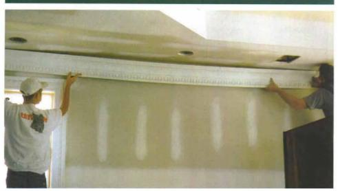
**Spring long pieces into place.** To make the seams disappear, butt sections are cut  $V_4$  in. long, glued up and sprung into place.
