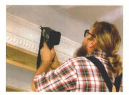
After the glue is applied, polyurethane crown is nailed up just like wood. To anchor the molding solidly while the adhesive cures, 8d finish nails are driven into the wall and ceiling framing.
