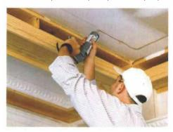
**Tracing lines for glue minimizes the mess.** A crew member runs out full-length  $V_4$ -in. beads of adhesive just inside pencil lines that denote top and bottom edges of the molding.
