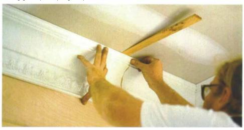
**Shim to align the faces.** Because molding thicknesses are inconsistent, a shim here and there is necessary to blend the faces where they butt together.
