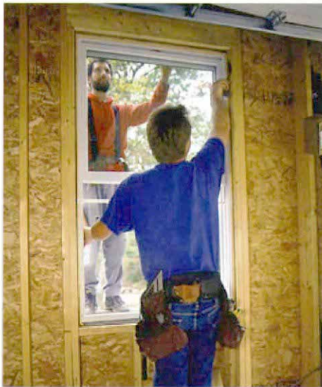
Center the window first. The outside crew member holds the window in place while the window is centered in its opening from the inside.
