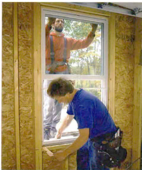
Two sides of window installation. A level is held outside on the head of the window (photo above), and instructions are given to the inside crew member to shim the window as needed (photo left).
