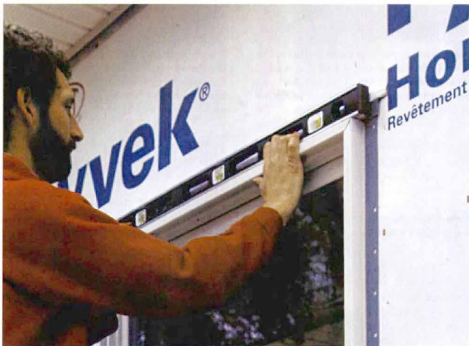
Two sides of window installation. A level is held outside on the head of the window (photo above), and instructions are given to the inside crew member to shim the window as needed (photo left).
