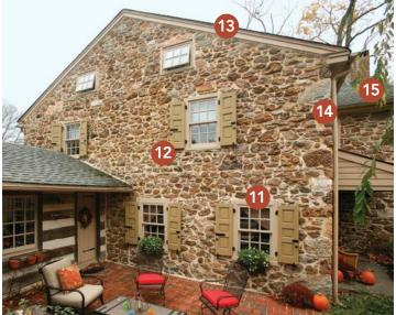
retrofitted into the masonry openings. Casings and jambs were sloppily packed in to make up any discrepancy in sizes. We selected wood replacement windows by Marvin with historically appropriate details and six-over-six divided lites. These windows enabled us to maintain the character of the home while taking advantage of their thermal performance. In addition, each window was custom-made to its specific opening for a tight fit.
