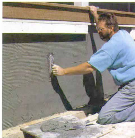
A textured finish provides better grip. A notched trowel creates a furrowed surface that is better for bonding the manufactured stone to the wall.
