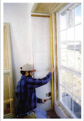
It's a rare house that is perfectly plumb and level. Shims make for a plumb and square nailing surface, and to ease placement, the author builds the floor-toceiling panels slightly short, hiding the gap with base molding.
