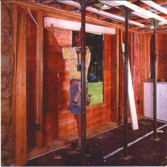
Header slides in first. A double 2x6 header is supported by the jack stud on one end and is tacked in place flush with the top of the king stud on the other end.
