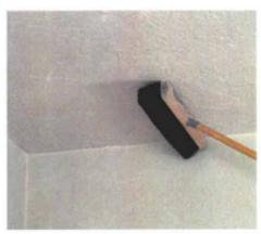
Wait a week before doing this. Scraping the wooden backside of a push broom over the dried texture knocks loose any fragile particles before they get caught in the paint roller.
