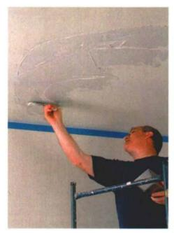
**One circle at a time.** Rather than take on the entire ceiling at one time, the author breaks the job into a series of overlapping circles. After quickly drawing an arc with a pencil, he begins by randomly slopping a thick layer of ready-mix joint compound within the confines of the circle.
