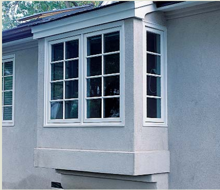
Sometimes you can build in the setback. This 2-ft. deep bay window was approved by the building department because it doesn't count as floor space. Photo taken at C on floor plan.
