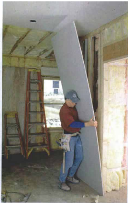
Tilt backward and lift from waist height to position a large vertical sheet.
