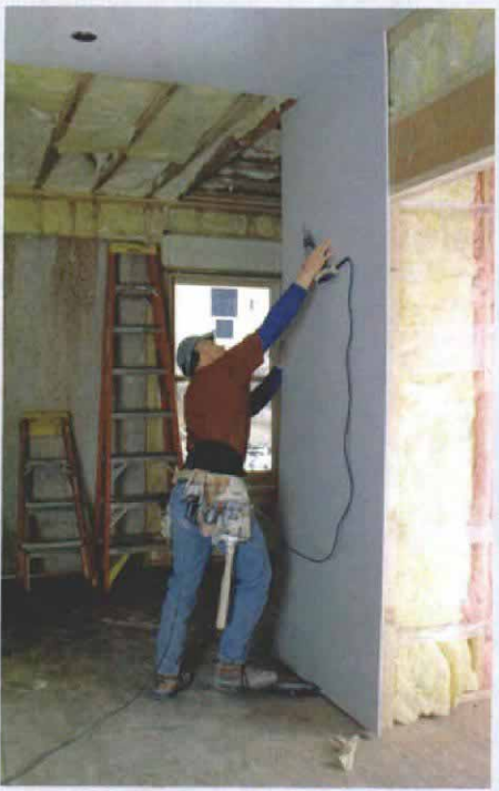
Steady the sheet with one hand until it's held tight to the ceiling with foot pressure.
