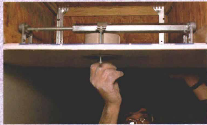
Specially designed ceiling box hangs from bracket.
