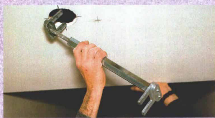
Remodeling bracket fits through a 4-in. hole.
